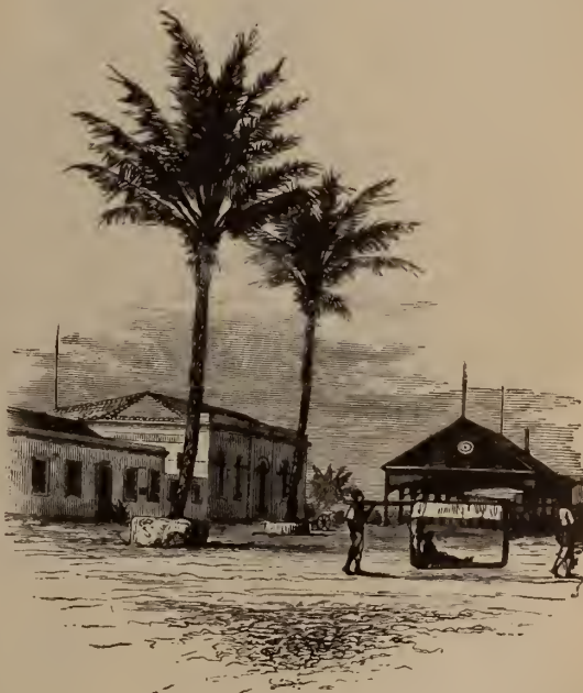
CUSTOM-HOUSE AT BENGUELA.
